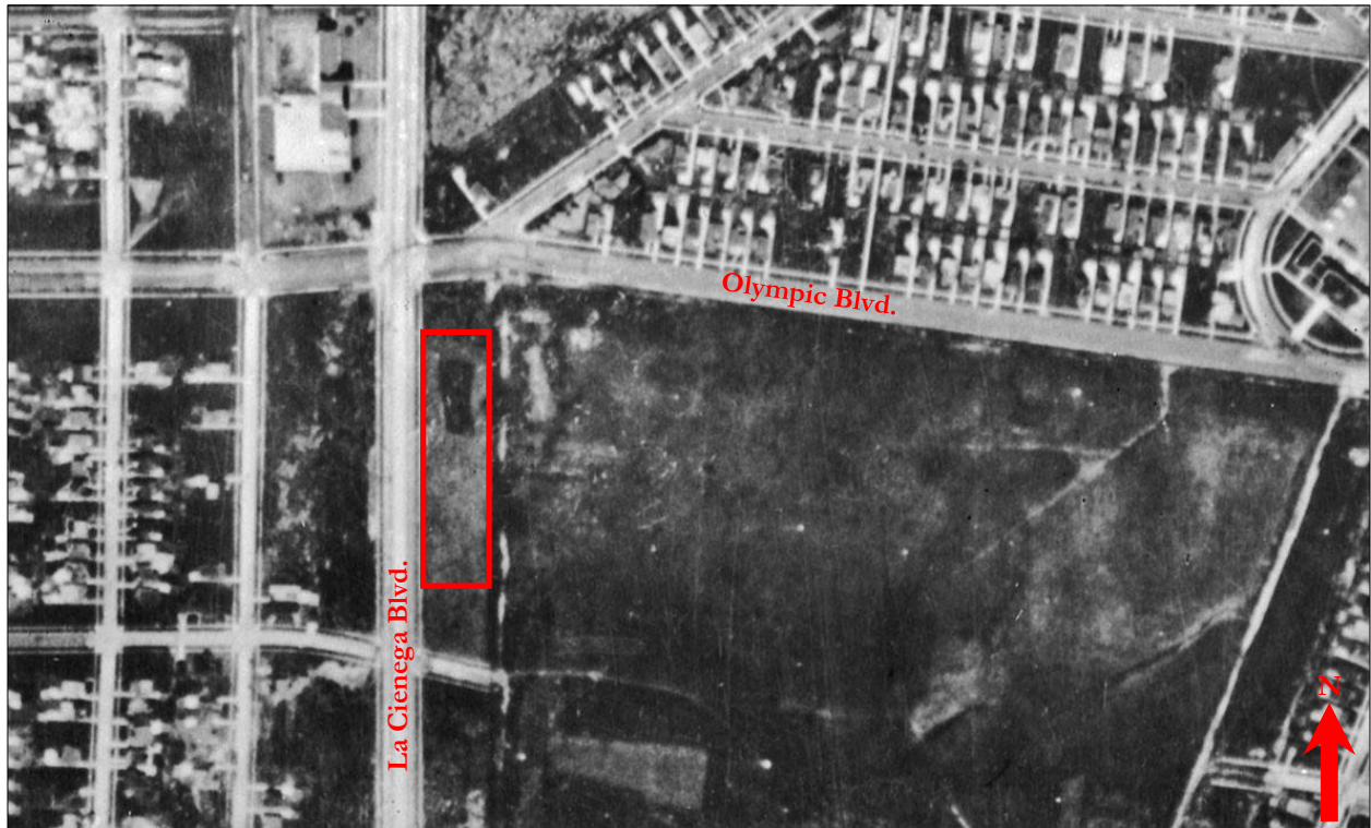
Historic Aerial 2: View north at the intersection of La Cienega and Olympic Blvd., approximate location of subject properties outlined (source: University of California Santa Barbara, 1928)
