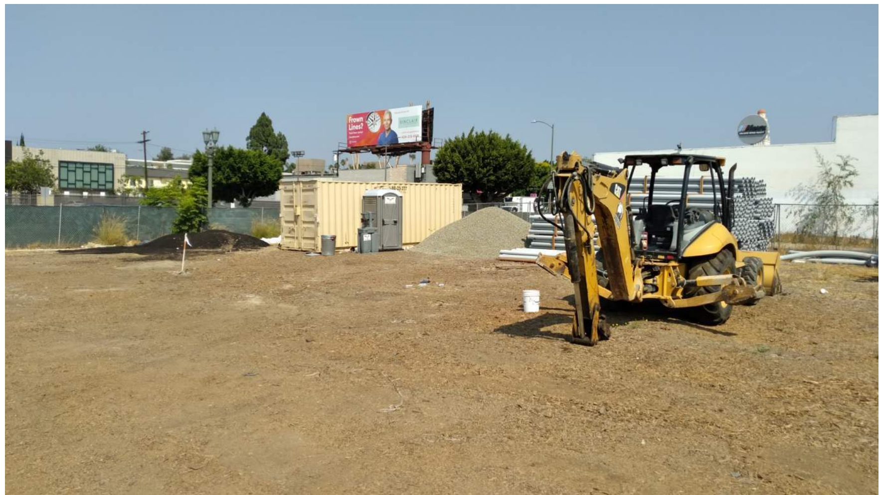
5 VIEW OF WEST SIDE OF SITE LOOKING NORTH
