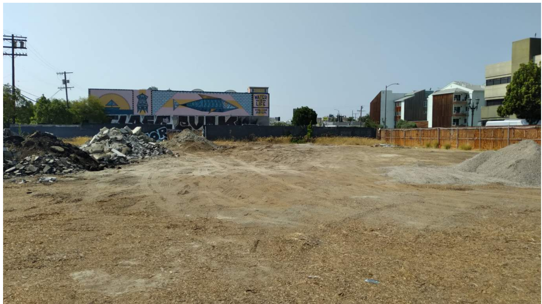
3 VIEW LOOKING TOWARDS SOUTH END OF SITE
